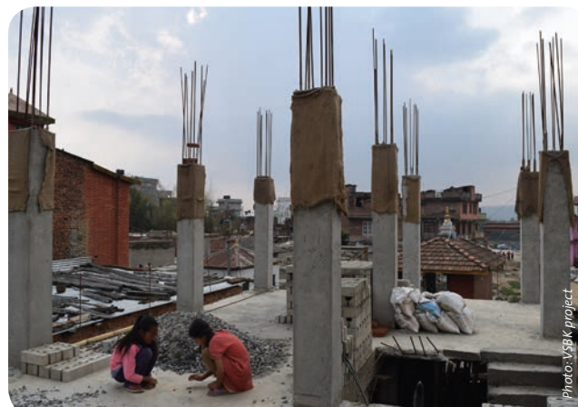
CSEBs are being used for Nepal's post-reconstruction efforts
