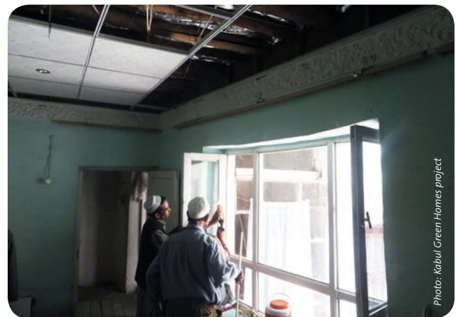
Double glazing and ceiling insulation installation
